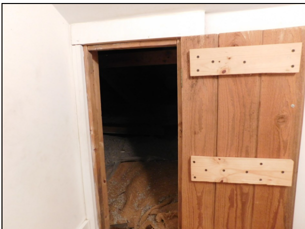
Access door to the hiding place within the attic
